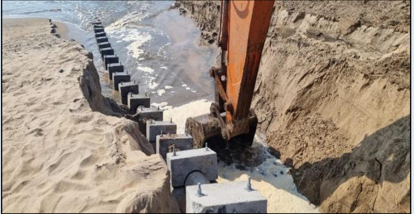
On-shore Burial of Pipeline
