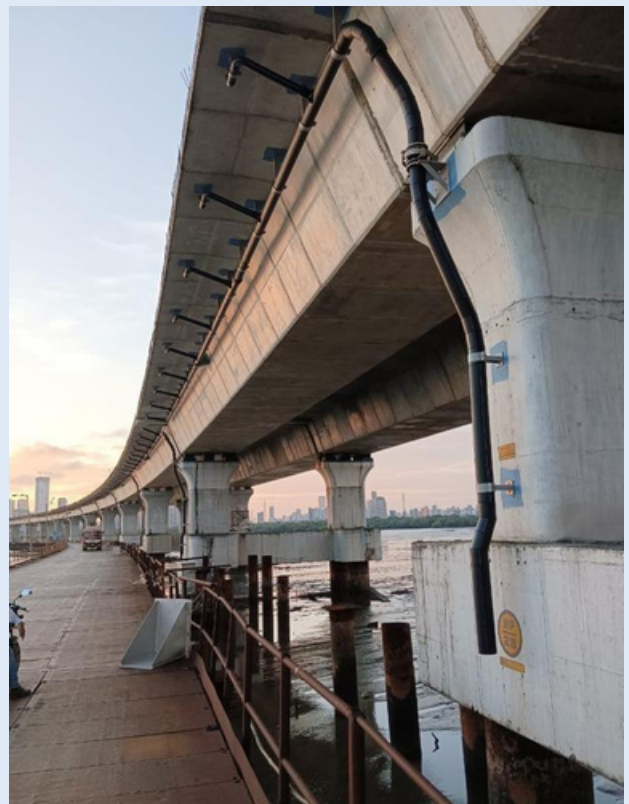
Span with Complete Pipes & Fittings
