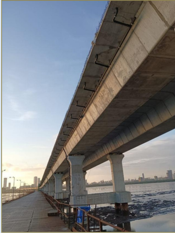
Different Views of a Span with Complete Pipes & Fittings
