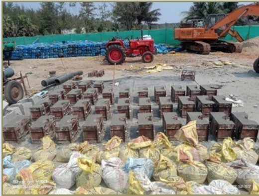
RCC Blocks Casting
