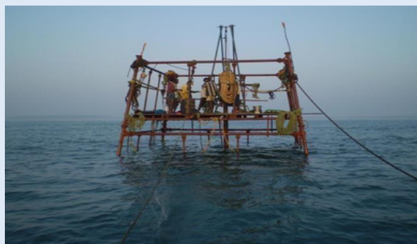
Platform Erection for Geotechnical Investigation
