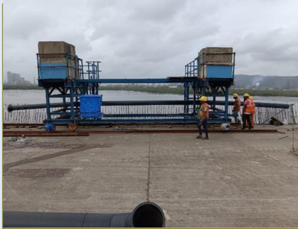
Pipe Installation using 'C' Platform
