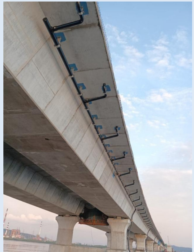
Different Views of a Span with Complete Pipes & Fittings
