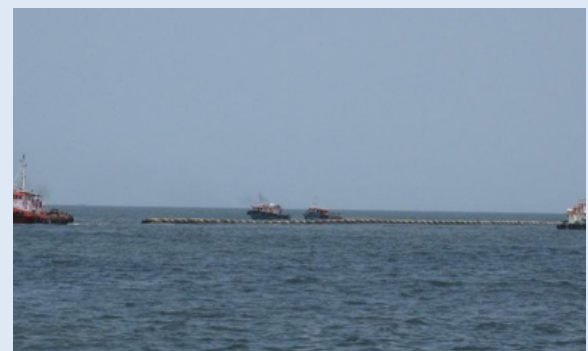
1600 mm OD Pipeline Towing in the Mid Sea
