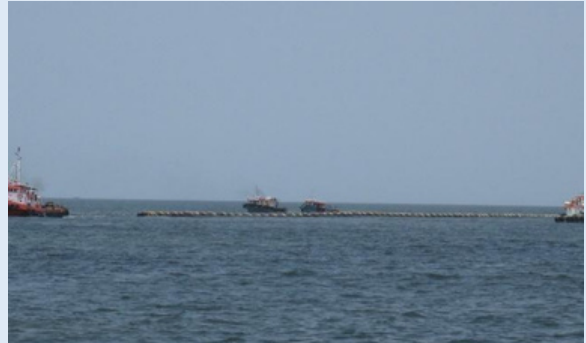
1600 mm OD Pipeline Towing in the Mid-Sea
