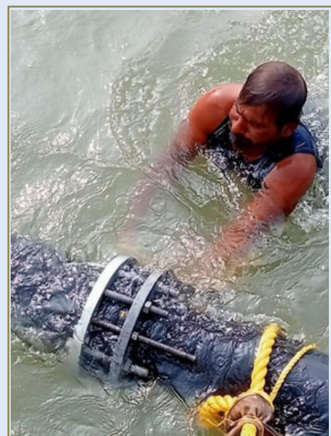
Flange Jointing of Pipes
