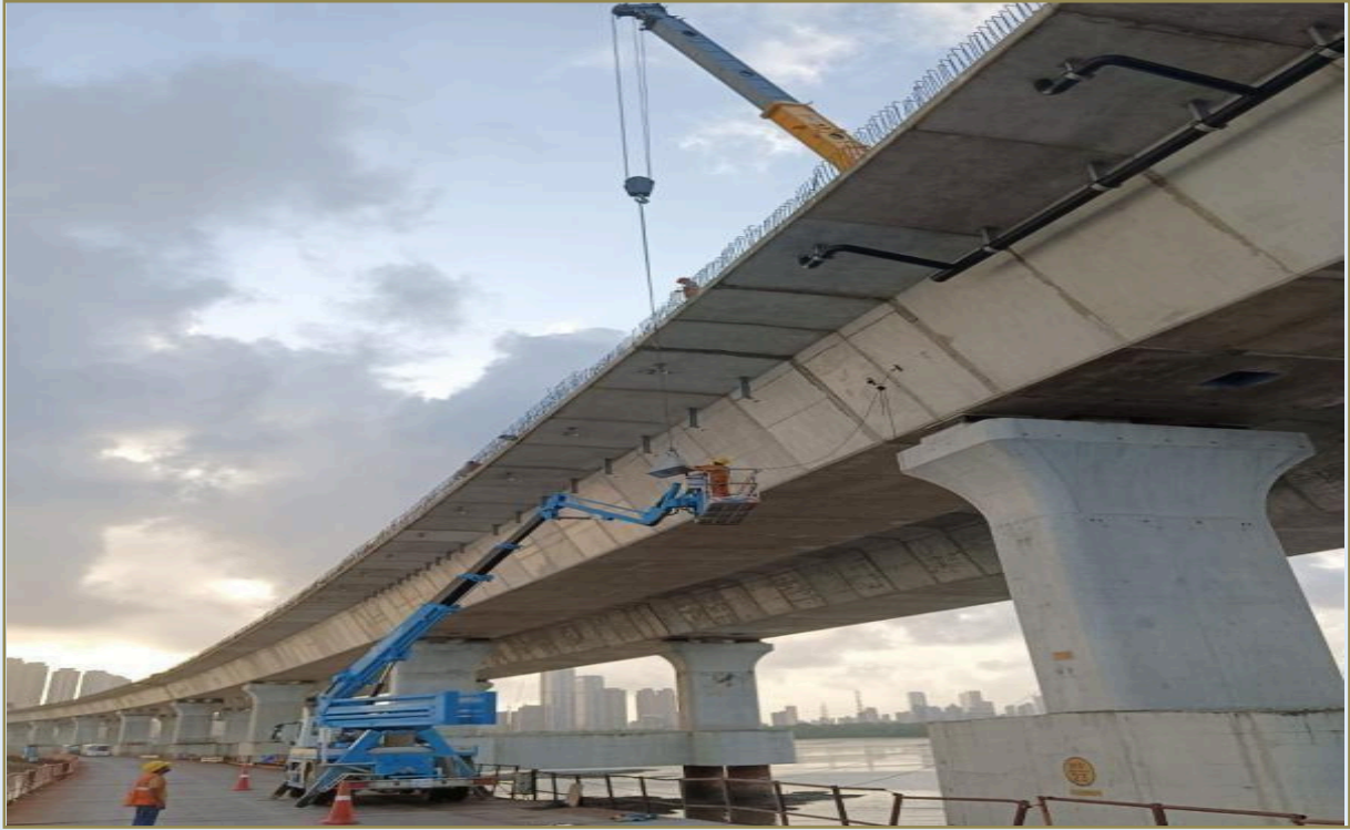
Guide & Anchor Support Installation
