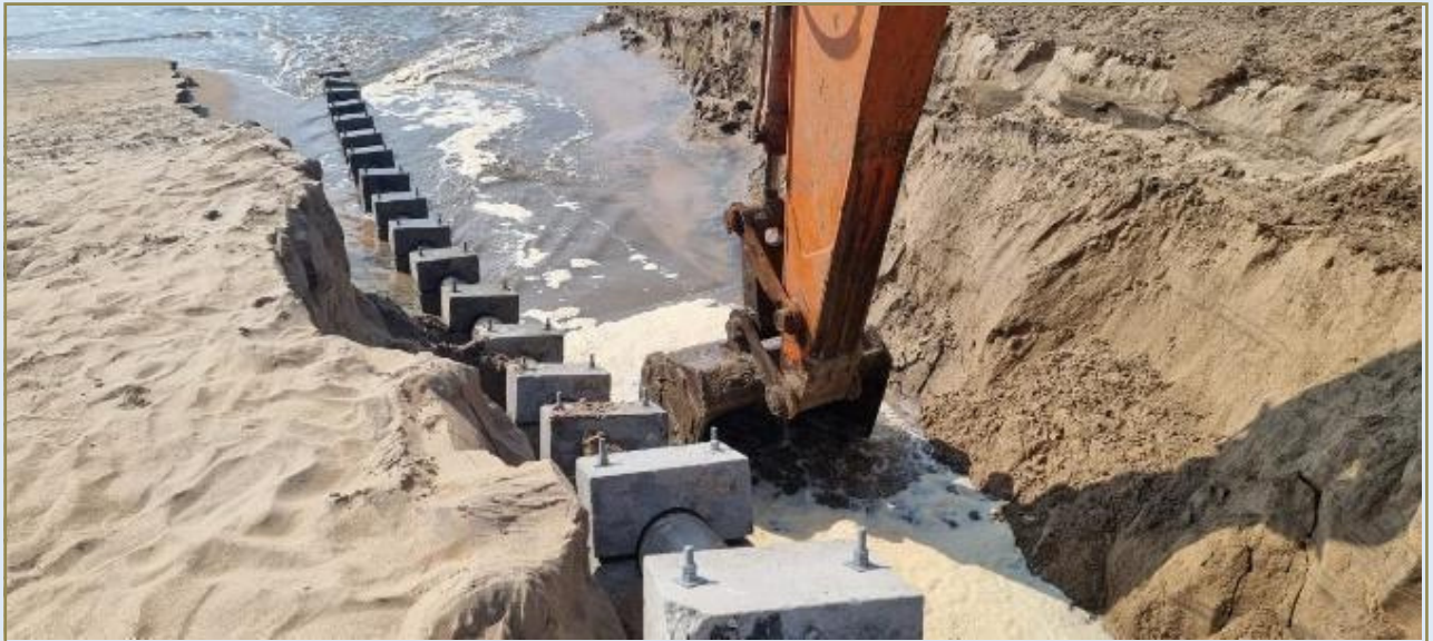
On-shore Burial of Pipeline
