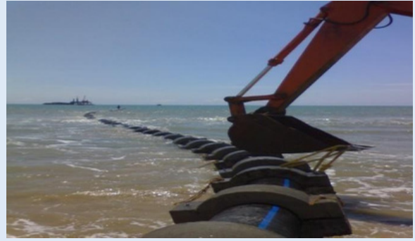
Pipeline Sinking in Process
