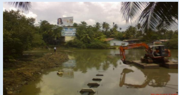
Pipeline Sinking in Trenches
