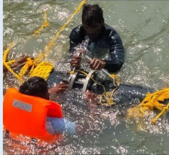
Divers Tightening the Bolts of Flange Jointing
