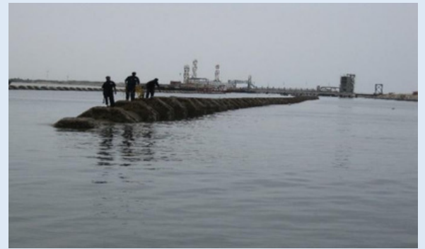
1600 mm OD Pipeline Sinking in Progress
