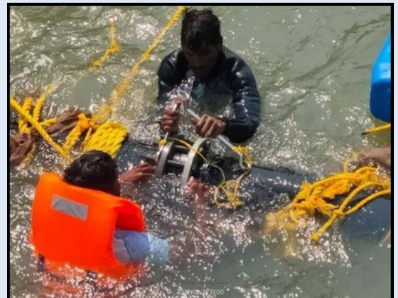
Divers Tightening the Bolts of Flange Jointing
