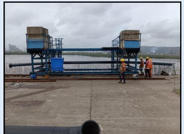
Pipe erection by using special designed platform
