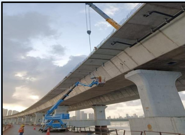
Guide & Anchor Support Installation
